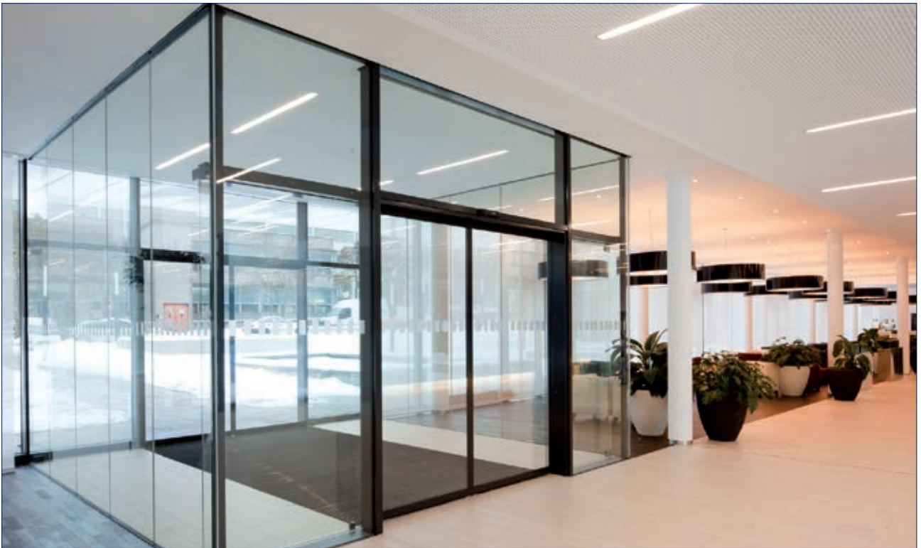
Slimdrive SL NT with vestibule, Augustinum, Stuttgart, Germany (photo: Dirk Wilhelmy)
