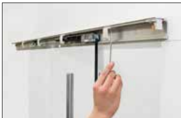
Mounting the clip-on cover bracket with the same Allen key
