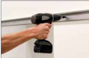
Attachment of the runner track from the front
